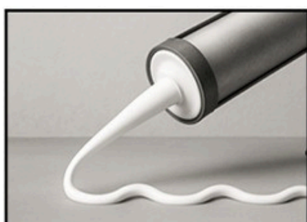
Apply the sealant in a straight bead to avoid gaps.
